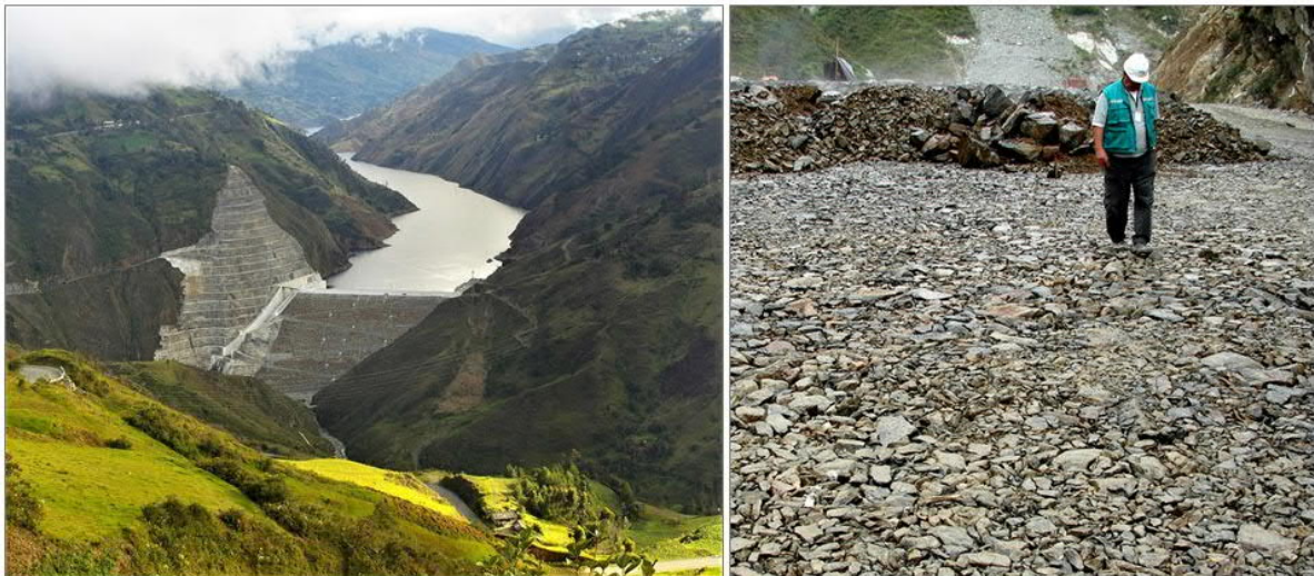
Figure 1 – A large rockfill dam, and the typical rockfill used for its construction
