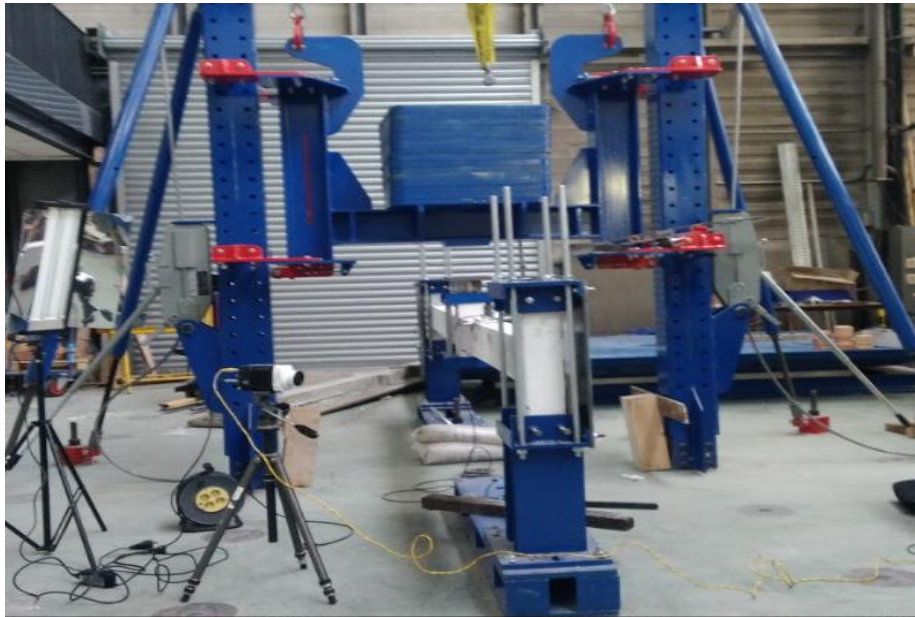
Fig. 3. Set-up used for testing beam-column subassembly under a middle column removal scenario
